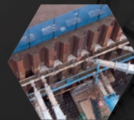
Trench Sheets & Sheet Piles
