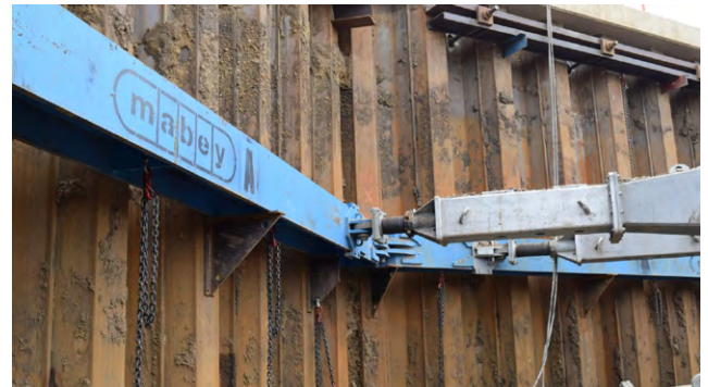
Mabey's Supershaft Plus system halved the installation and removal time of works at Kirkthorpe
