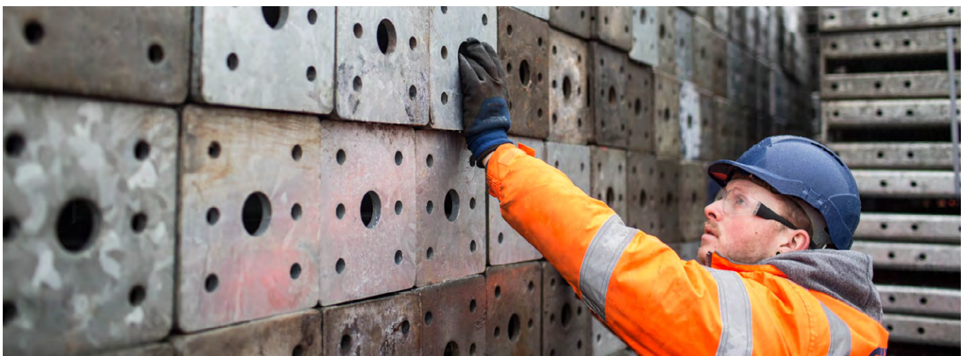
Mabey engineer on site in its Garswood depot
