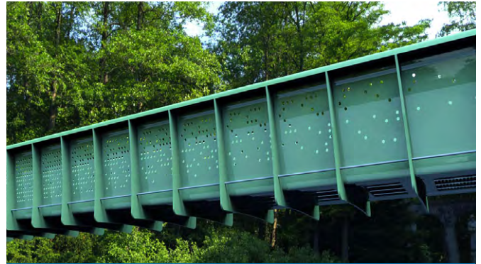
Mabey and Arup deliver the first rapid assembly, polymer, modular bridge
