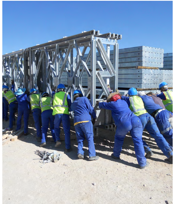
Engineers and locals join forces to build a bridge in Namibia
