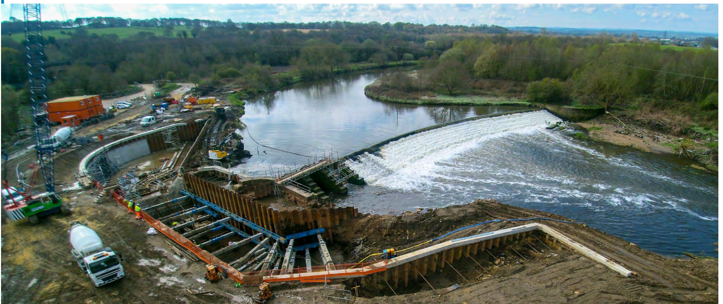
Aerial view of Mabey's propping system in Kirkthorpe
