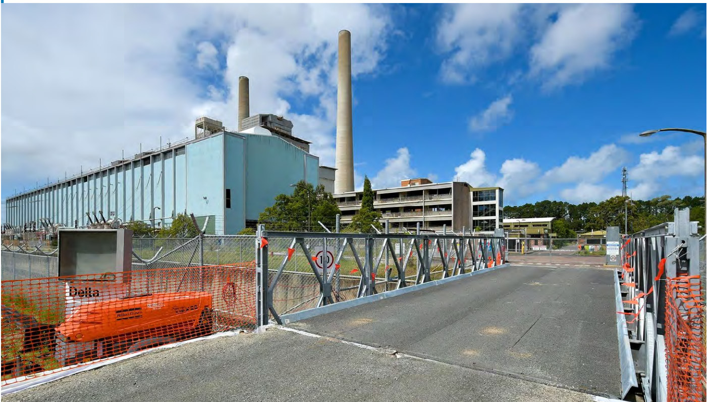
Mabey's Compact 200 (C200) bridge at Colongra Power Station
