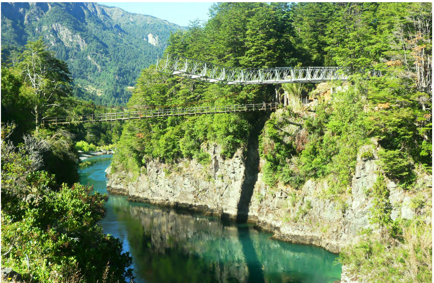
Mabey's C200 bridge being installed over a river in Chile
