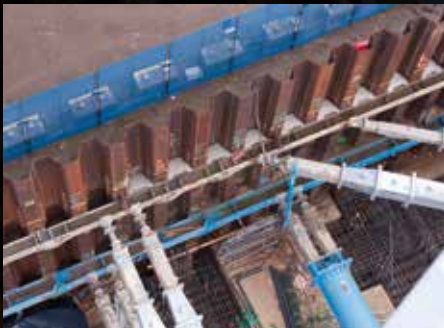
Trench Sheets & Sheet Piles
